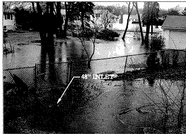
Photo 9: 48" CMP at Leitha Drive swale flooding during March storms, C&C March 2010
