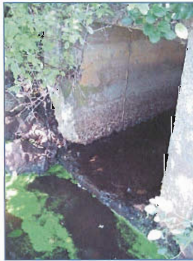
Photo 12: 36"x42" Reinforced Concrete Pipe outlet to Hardy Pond, C&C September 2010
